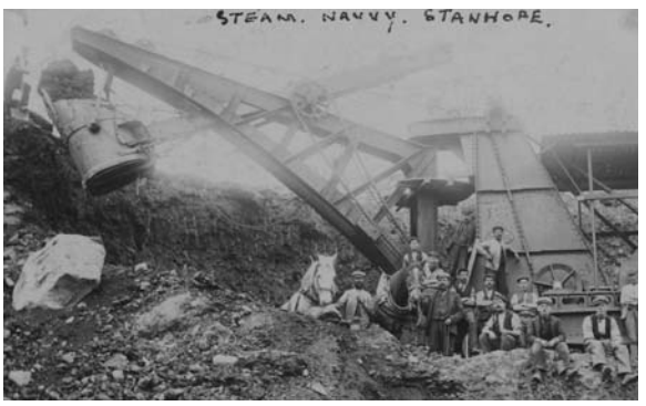
An old 'steam navy' removing the overburden. It required two drivers, a fireman, a banksman – 'to keep things right' – and horsemen.
